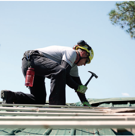
A Greyshirt tarps a roof in Coffee County, GA, damaged by Hurricane Helene.
